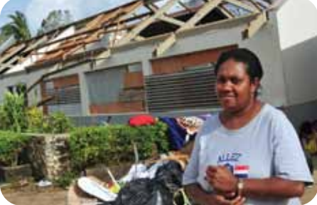
THE PRINCIPAL OF VILA NORTH SCHOOL OUTSIDE A BUILDING THAT HAS LOST ITS ROOF
