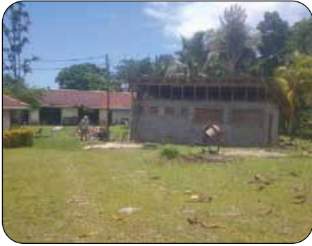
ABLUTION BLOCK, TALUA
